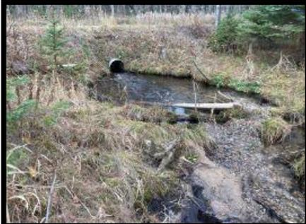
An undersized and perched culvert on a tributary of the Black River at Johnson's Crossing will be replaced with a larger culvert to allow trout to access upstream habitat.
