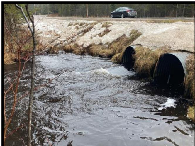
The existing crossing of the Black River at Sparr Road consists of two pipe culverts that are severely undersized for the stream, causing a choke point in the river and contributing to erosion and seasonal flooding. Huron Pines will install a much larger bottomless arch culvert to reconnect that stretch of river.
